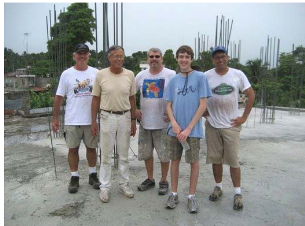
Team III men on newly poured roof.
