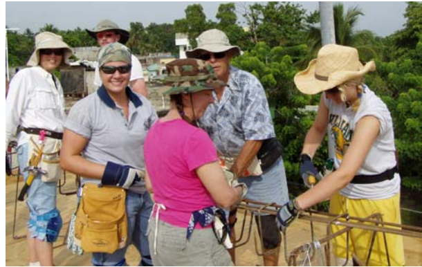
Team II members tying rebar
